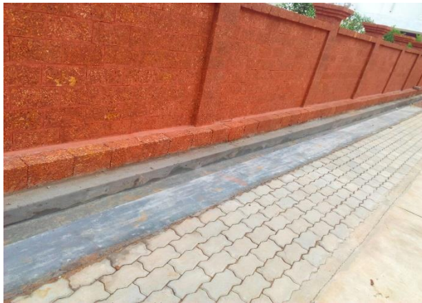
Compound wall Swarna Baharath Trust ,Vijayawada Arc Mahendra Kumar, Andra Pradesh
